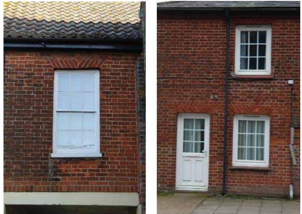
Figure 64 Examples of 'V' shaped red brick lintels
