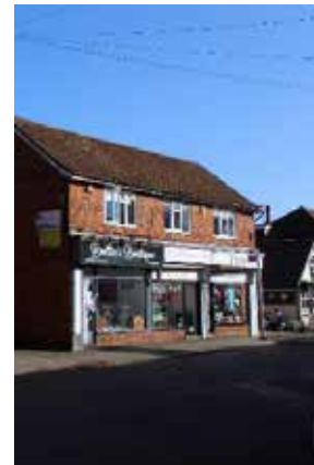
Figure 75 Modern Shop Front
