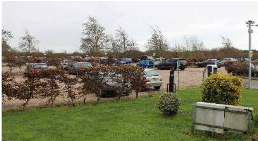
Figure 14 The Lifehouse Spa car park
