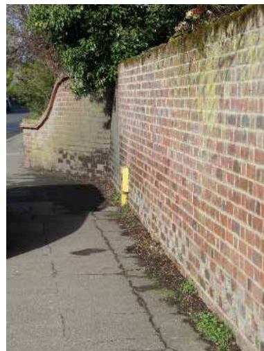
Figure 49 Flemish bond brick-built boundaries contribute to the character of the Conservation Area
