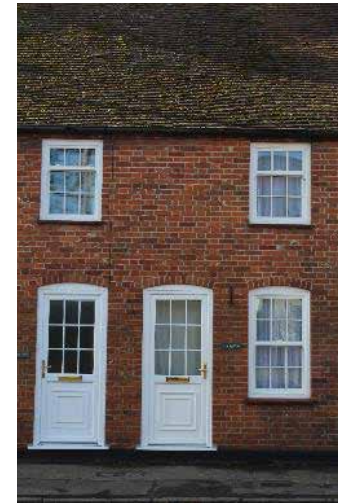
Figure 76 Loss of Architectural Details
